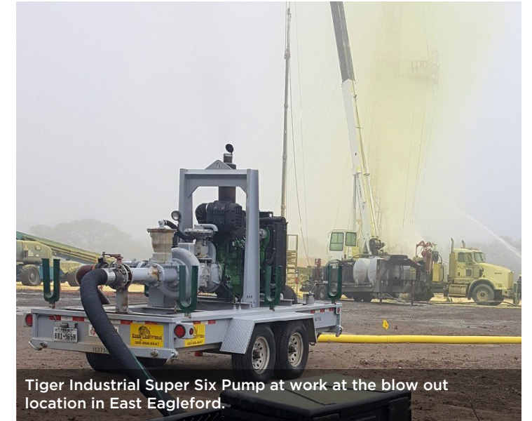
Tiger Safety Hydraulic Choke Package on East Eagleford blow out jobsite.
