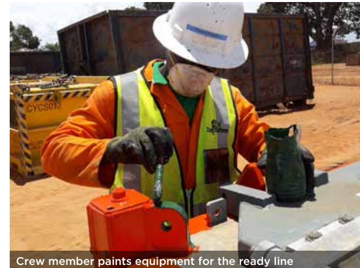
Crew member paints equipment for the ready line
